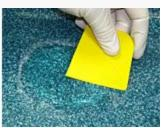
Repeat the filling process if grinding was too severe (see Granite repair procedure in website), and reapply the granite color application followed by grinding and sanding. The surface is now ready for the protective clear coat application. The final finish should be sanded with 220 grit wet or dry sandpaper.
