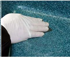
Wipe the surface clean using isopropyl alcohol and paper towel or a clean cloth. Dry or wet sand the grinding marks using 100 or 220 grit, wet dry sand paper. Wipe the surface dry and repeat the isopropyl alcohol application if necessary.
