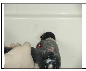
1) Prepare the damaged area, crack or break from the cosmetic surface side first. Grind out the cracks and damage to fit the repair area back to its original shaped form. This can be achieved by grinding the cracks with a disc set-up on a drill, dremel tool or by cutting with a utility knife or small saw if necessary.
